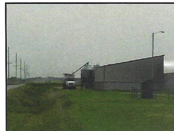
Drive and park in designated areas. Follow all posted signs.
